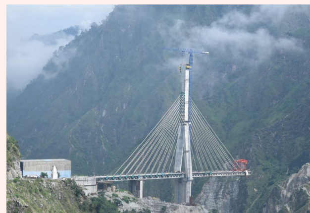
Tallest Cable bridge 331m over Anji river in J&K for Rail & Road
